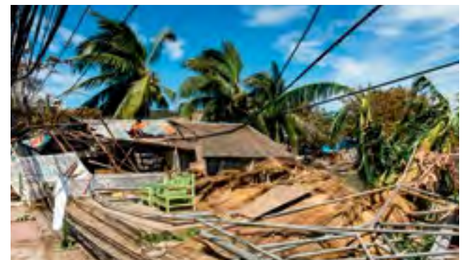
A wooden building reduced to rubble by Super Typhoon Haiyan
