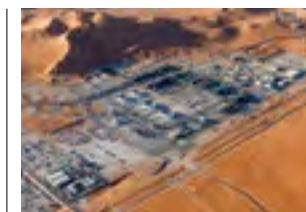
The El Merk facility, Algeria
