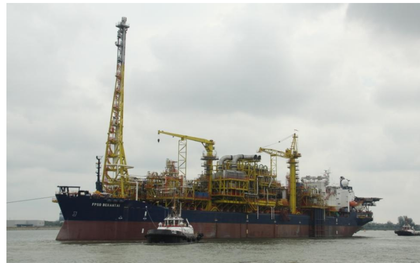
FPSO Berantai, Malaysia
