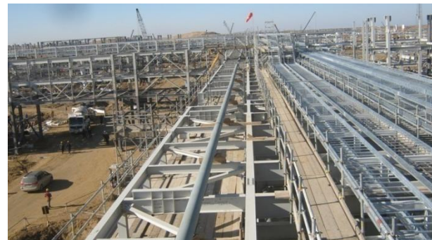
South Yoloten gas field development, Turkmenistan
