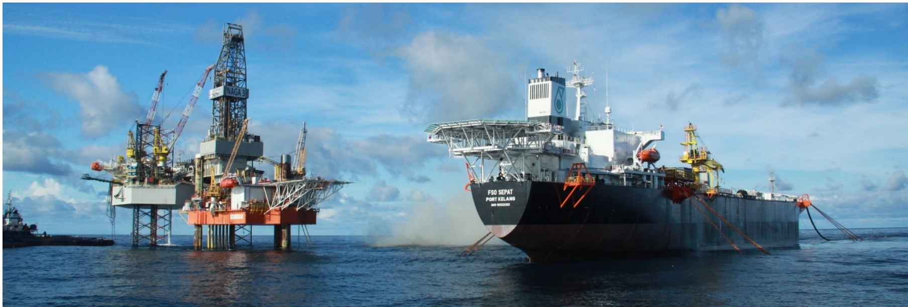
SEPAT offshore early production system, Malaysia
