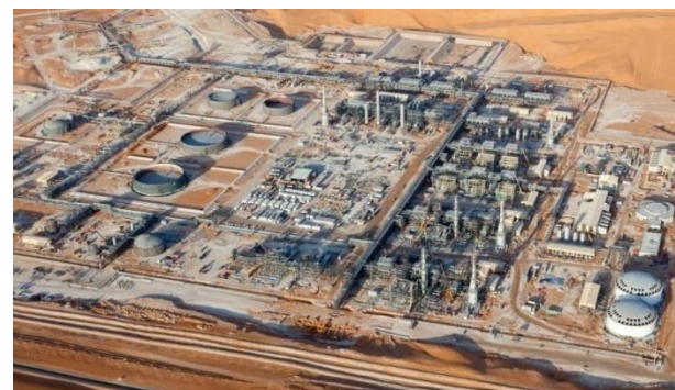
El Merk gas processing facility, Algeria
